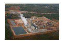
Project utilizes approximately 500,000 tons of woody biomass annually, consisting of urban wood waste, mill and logging residues. Piedmont qualifies as a source of renewable power under federal and state standards.
